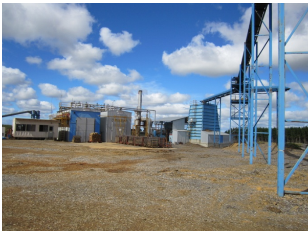
Figure 15: The current sawmill residue management and boiler system providing heat to kiln dry green sawn timber prior to subsequent value adding.
